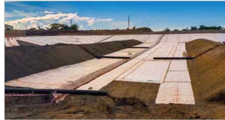
7,00,000 sq. m. Ecoklay LWP Landfill Project, West Papua, Indonesia
