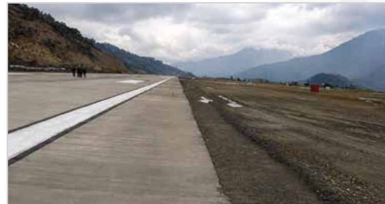
1,80,000 sq. m. Geoklay 350 Runway Project, Pakyong, Sikkim Airport
