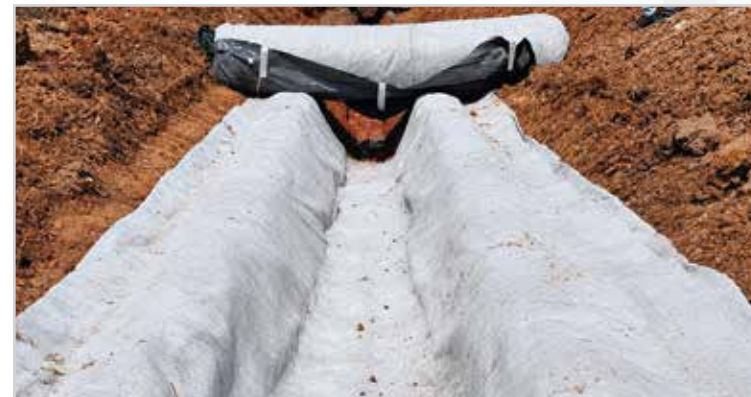
15,000 sq. m. Cretematt Railway Project, Rahul Kela, Odisha
