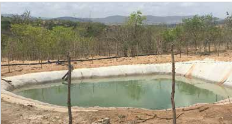
4,000 sq. m. Pond Lining Project, Munnar, Kerala
