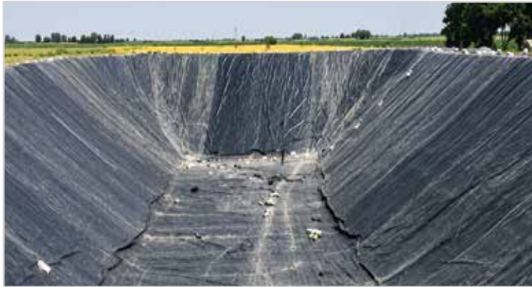
4,000 sq. m. Ecoklay LWP Pond Lining Project, United Arab Emirates
