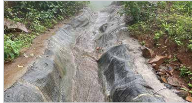
10,000 sq. m. Creteroll Rain Water Catch Drain Canal, Project, Igatpuri
