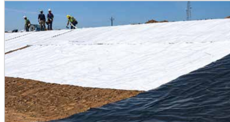
1,00,000 sq. m. Ecoklay LWP Landfill Project, Malaysia
