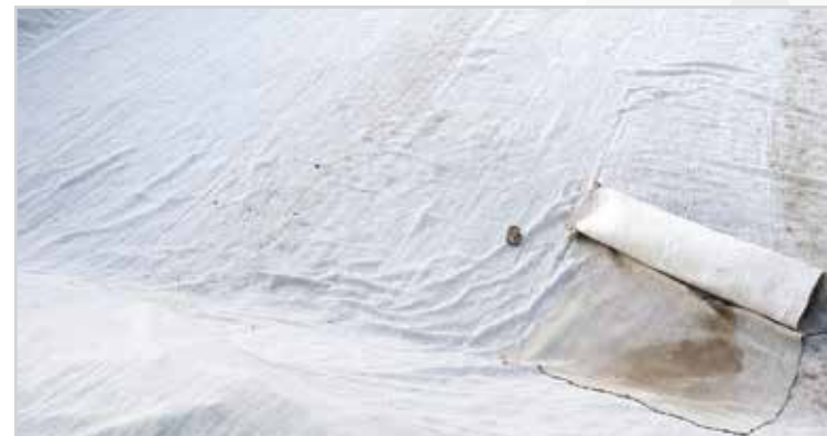
10,000 sq. m. Ecoklay SPL Pond Lining Project, Belgium
