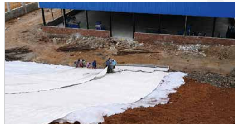
6000 sq. m. Pond Lining Project, Munnar, Idukki District, Kerala
