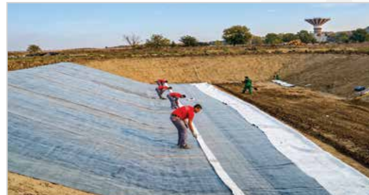
6,800 sq. m. Ecoklay SPL Land Filling Project, Colombia
