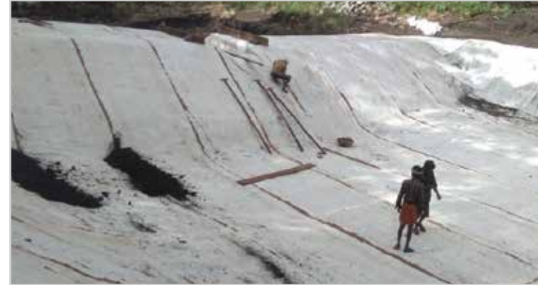
3,000 sq. m. Koviloor Check Dam, Soil Conservative Project, Kerala
