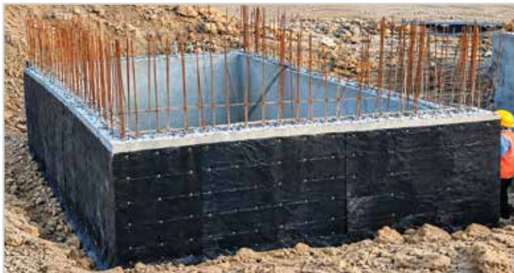
Ecoklay LWP, Basement Waterproofing Project
