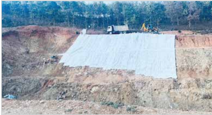
19,000 sq. m. Mining Operations Cretematt Project, Surjagar Hills, Etapalli, Gadchiroli, Maharashtra
