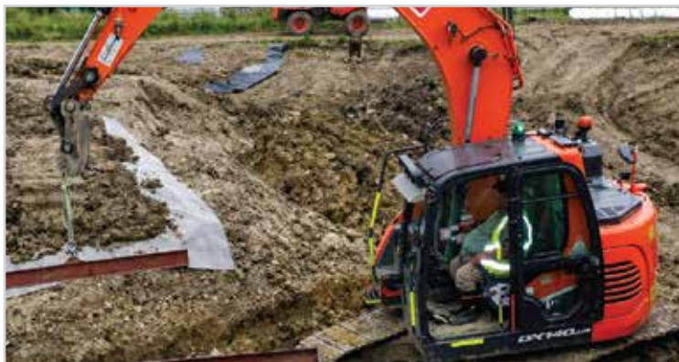
8,000 sq. m. Ecoklay LWP Pond Sealing Project, United Kingdom
